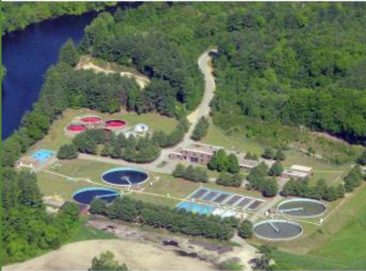
Franklin wastewater treatment plant
